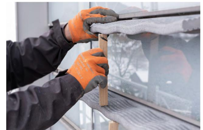
AUSRICHTEN, TROCKNEN - UND FERTIG IST DIE 3D.SOLAR-FASSADE
